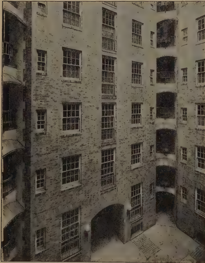
691 Henry Atterbury Smith, architect; photograph by Wurts Brothers
